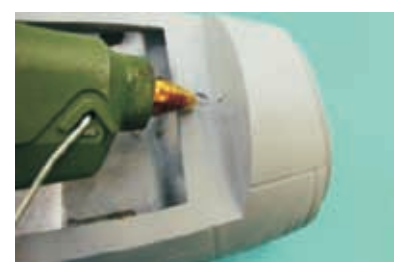
11.12 Apply foam safe hot glue in the slot.
